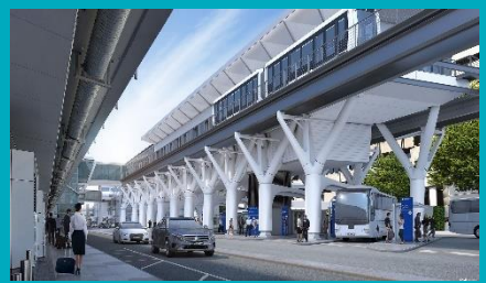
Neue Sky Line Station vor Terminal 1
